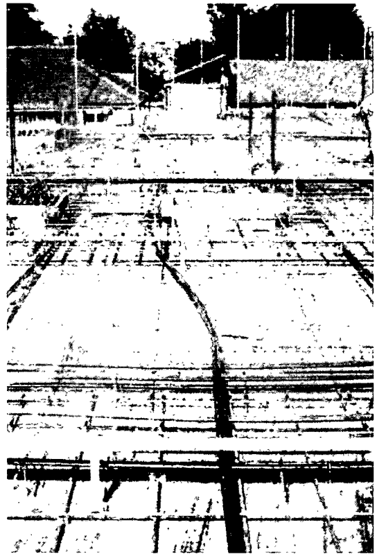
Figure 53: Unbonded tendons diverted around an opening.
