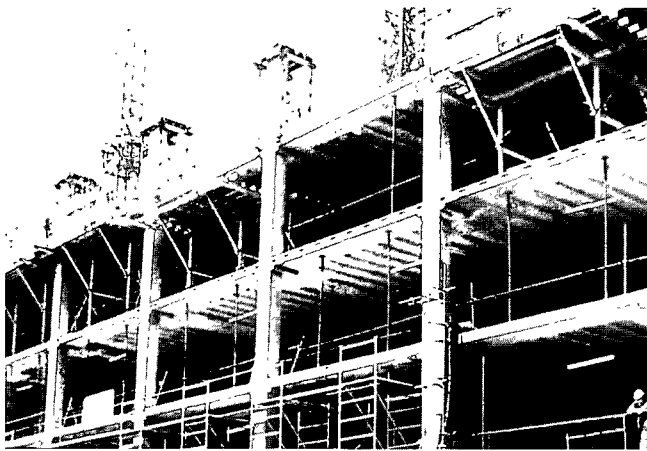
Figure 6: Post-tensioned ribbed slab.
