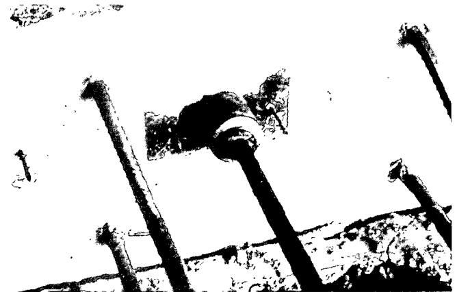
Figure 54: Intermediate anchor at construction joint.
