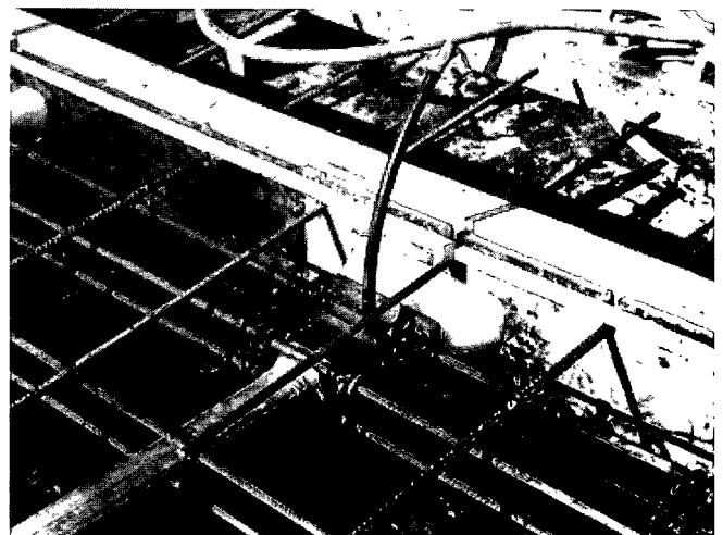
Figure 62: Anchorages for bonded tendons: fixed to formwork.
